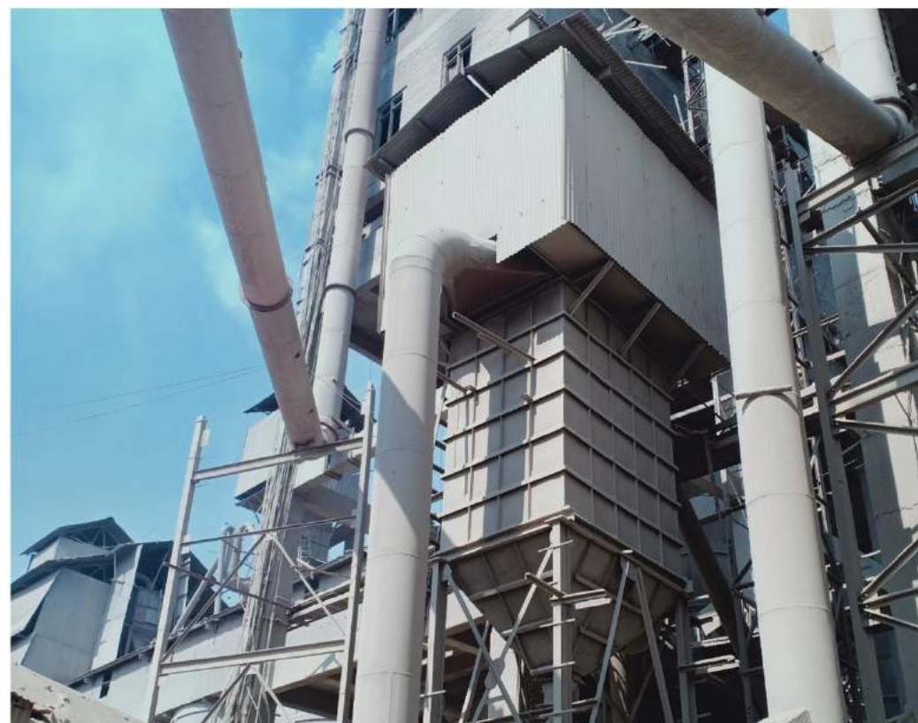
Fig.-1.8 Dust collectors attached to Clinker crusher
