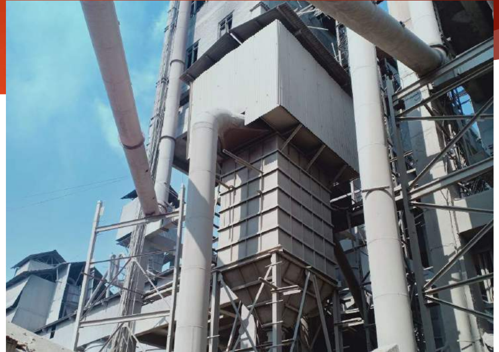
Fig.-1.8 Dust collectors attached to Clinker crusher
