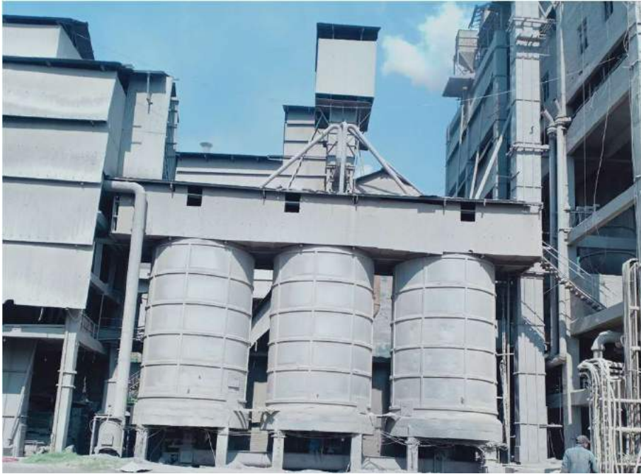
Fig.-1.19 Silos with bag filters
