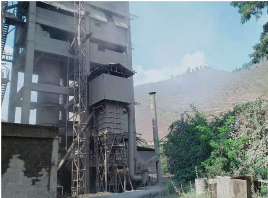
Fig.-1.9 Dust collectors installed
